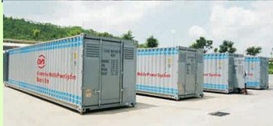
20# container 250kW/250kWh
