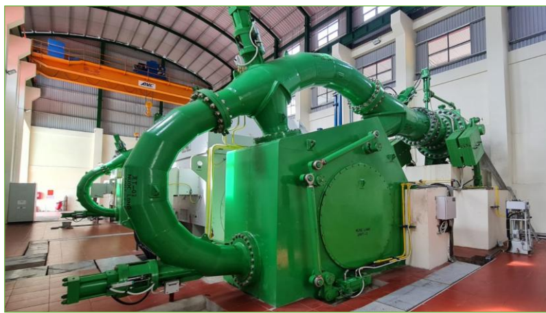
NUOC LONG HPP : Horizontal 3 jet Pelton 2 x 15MW = 30MW Head: 530m Commissioned in 2022, at Vietnam
