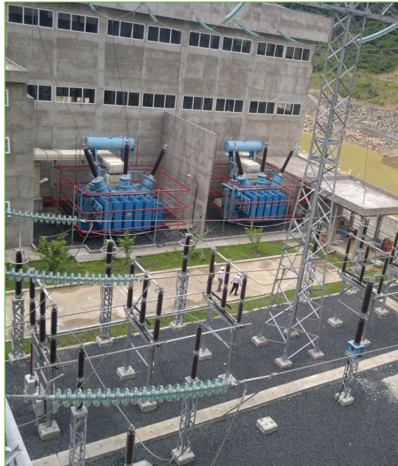
SONG BUNG 4A : Vertical Full Kaplan 2 x 27MW = 54MW Head: 33.2m Commissioned in 2014, at Vietnam
