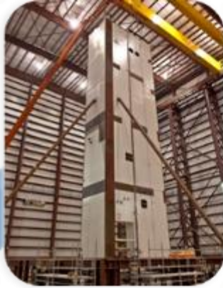
Factory production of modules
