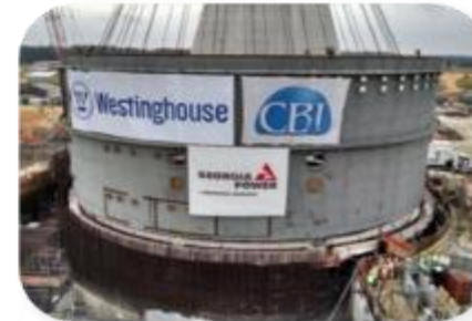
Construction and module assembly
