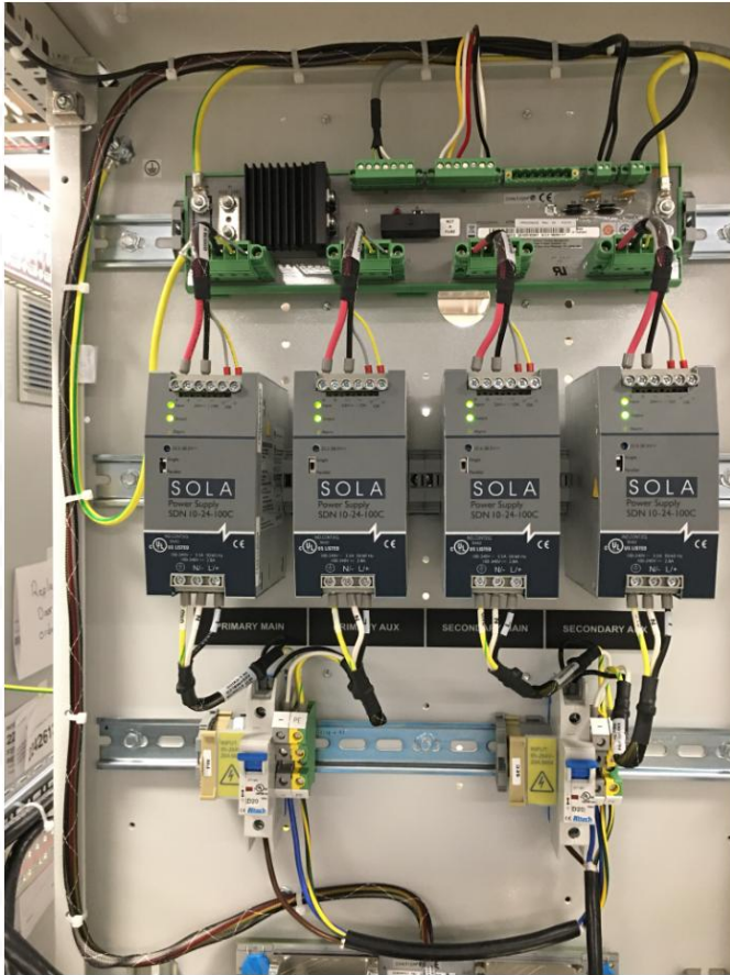
Redundant Power Supplies
