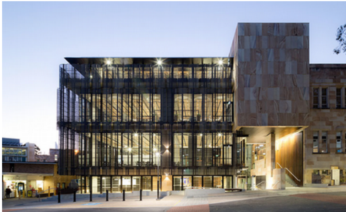
Queensland's University GCI building with 3 suspended floors made from structural geopolymer concrete
